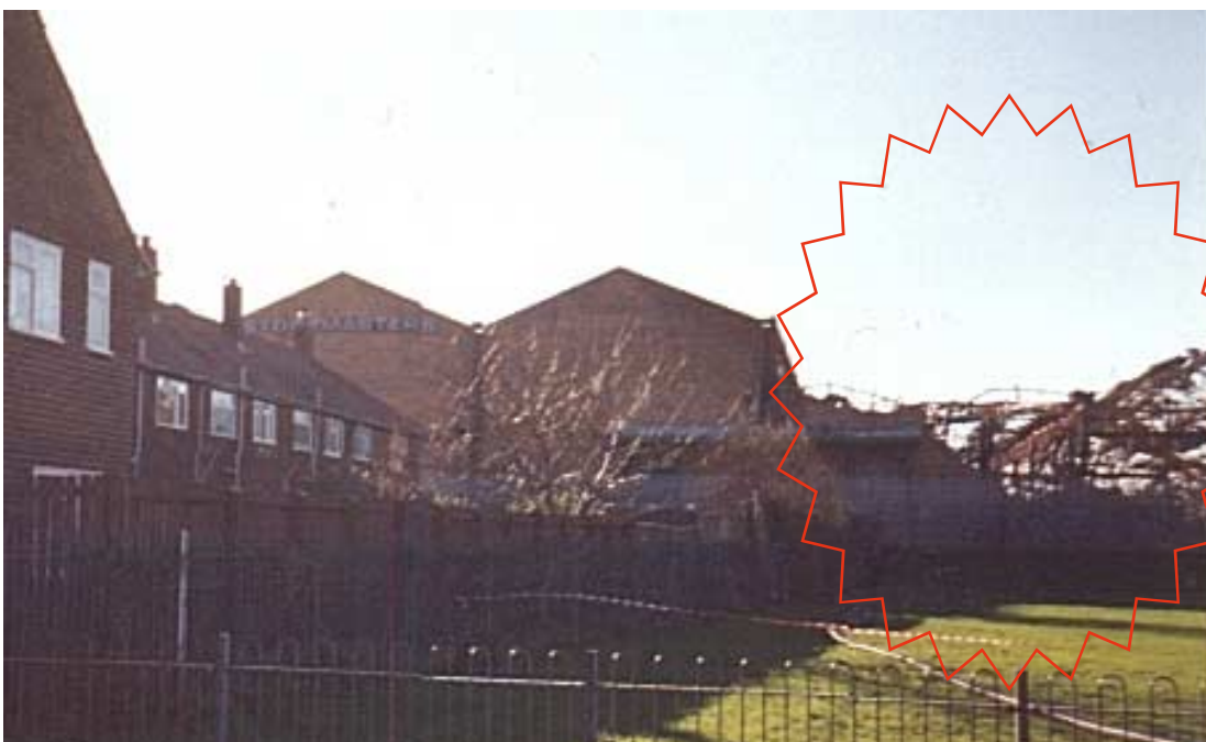
Photograph 1: Proximity of warehouse to housing estate and primary school © Fiona Welch, CIRS
