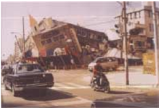
Photograph 1: Example of collapsed buildings in Kobe (Kristin Hanson)
